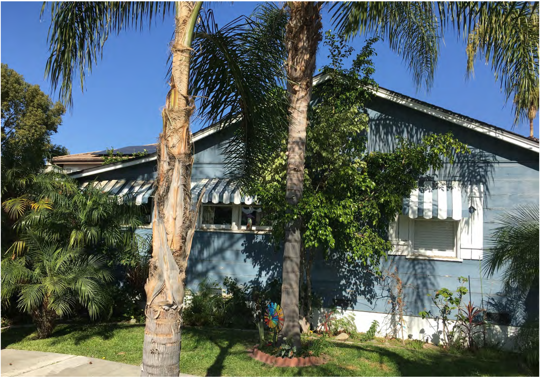
PHOTO - SOUTH SIDE - FANO STREET
